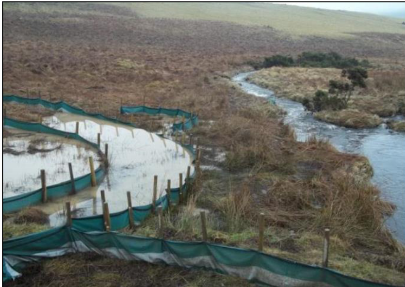
Plate 5.1: Photograph of Silt Fencing
