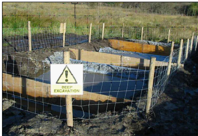
Plate 5.2: Completed Settlement Pond System
